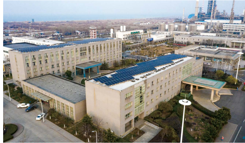
Rooftop photovoltaic modules at the Qingdao Refinery and Chemical Complex
