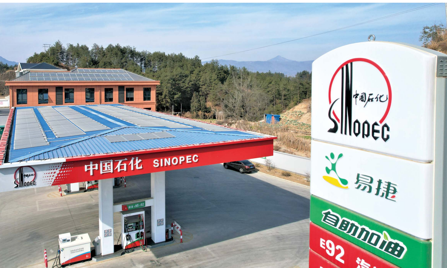
⚡ Rooftop photovoltaic power generation unit at Jiaze refuelling station in Changzhou, Jiangsu generates 127,000 to 147,000 kWh of electricity annually
