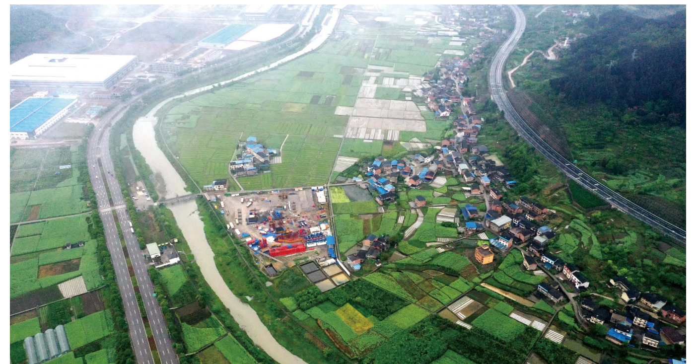
④ Huadong Petroleum Engineering Company's Shengye 2 platform minimises land use during the construction process
